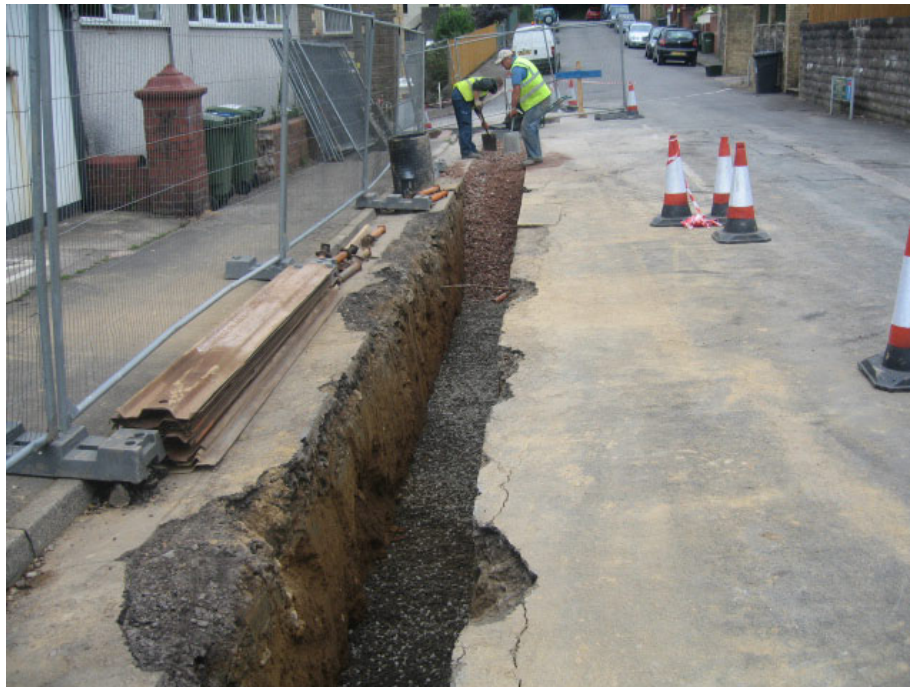
Trench through carriageway
